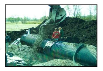
Backfill must be placed and fully compacted to the minimum cover level over the structure before the pipe is subjected to highway or light construction loads.
